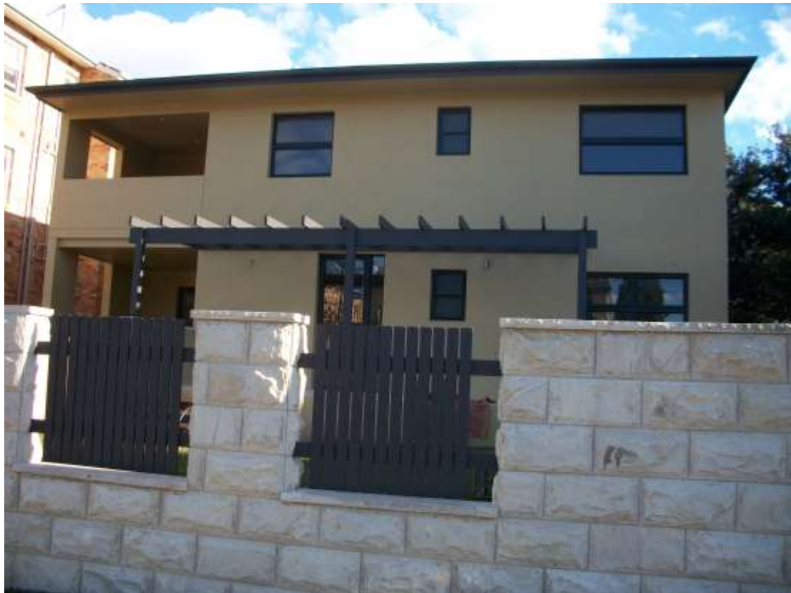
Building still under construction at No. 19 Moore Road, Freshwater
