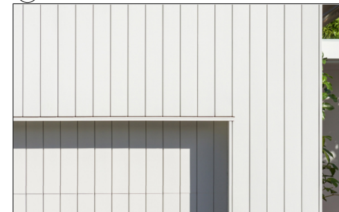
B VERTICAL WHITE EXPRESSED CLADDING
