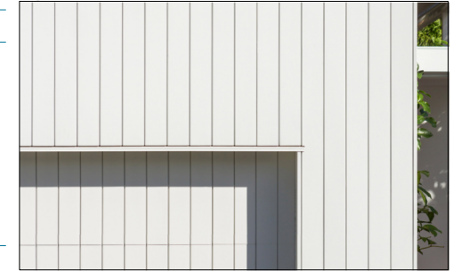
B VERTICAL WHITE EXPRESSED CLADDING
