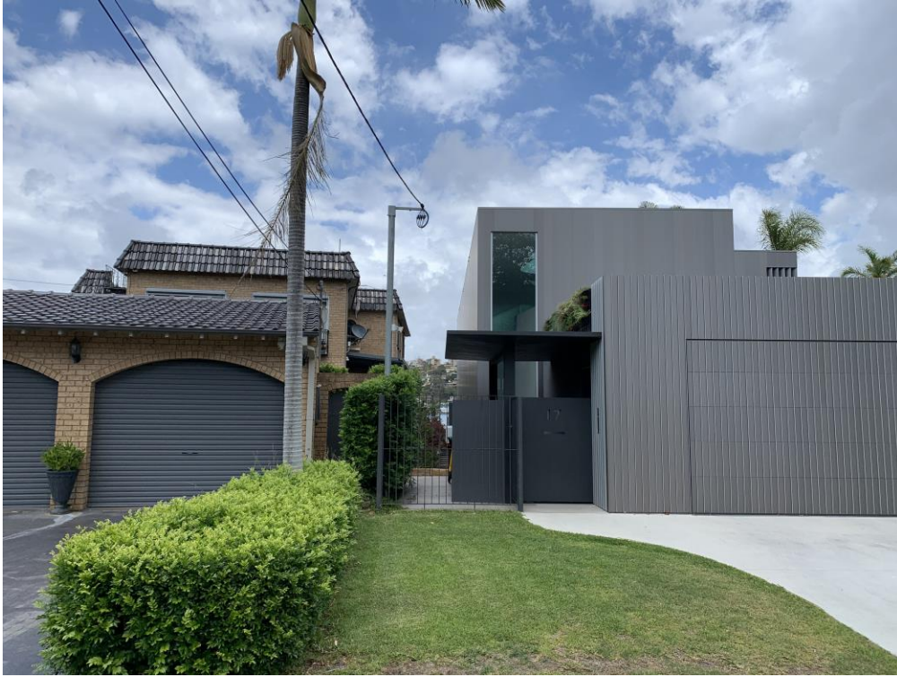
Fig 6: View of subject site and neighbouring dwelling at No 17 Monash Crescent, looking south-west
