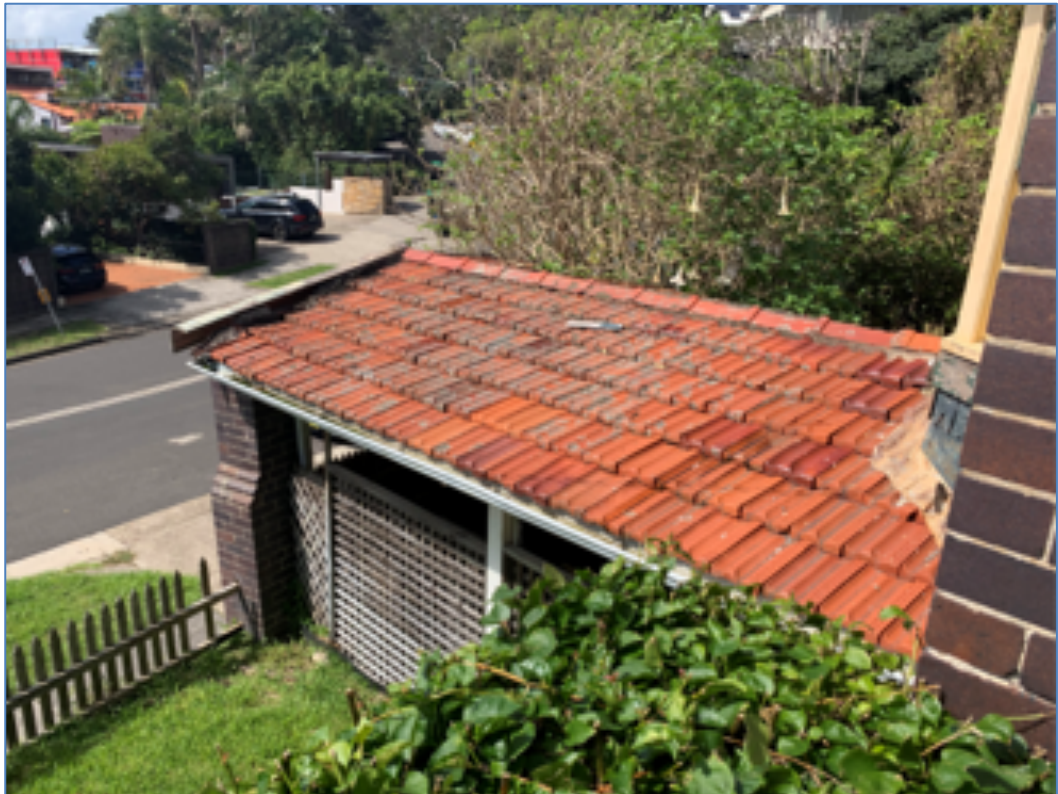
Figure 8: View to the front carport structure from the front balcony.
