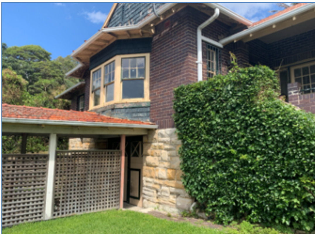
Figure 5: View to the front carport and front gable from the front lawn.
