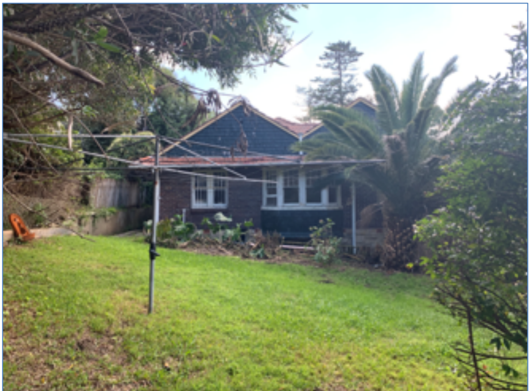
Figure 7: View to the rear elevation and the rear of the garden.
