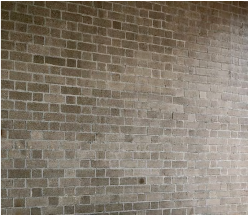
brick walls at base
