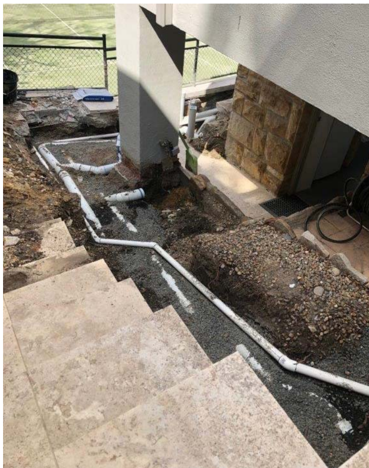
Image 3 looking south showing extent of plumbing repair work
