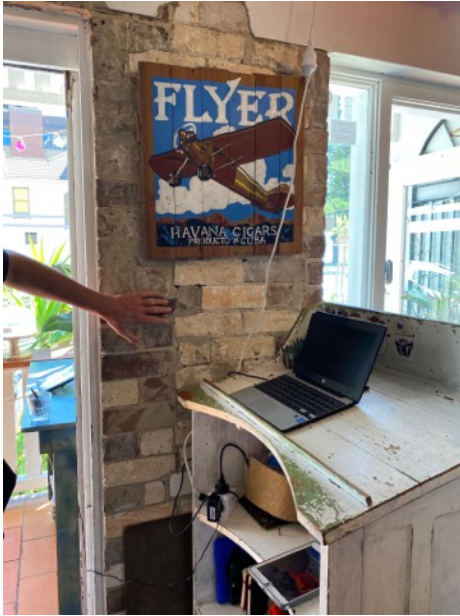
Figure 24.0, Render removed from brickwork, AW 2020
