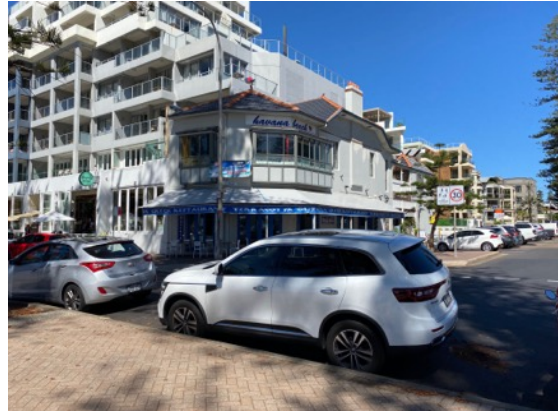
Figure 15.0, Corner Victoria Pde and South Steyne, AW 2020
