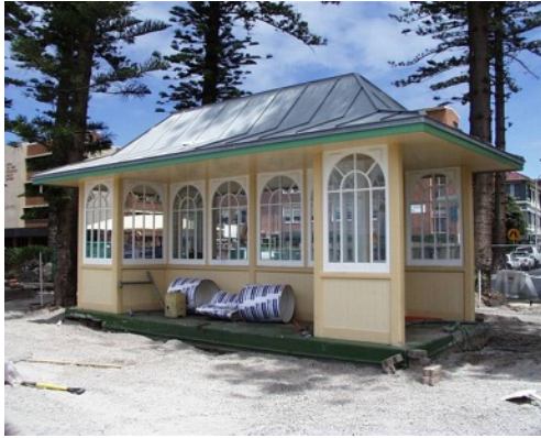
Figure 43.0, Public Shelter's (2) Federation. South Steyne. Environment NSW
