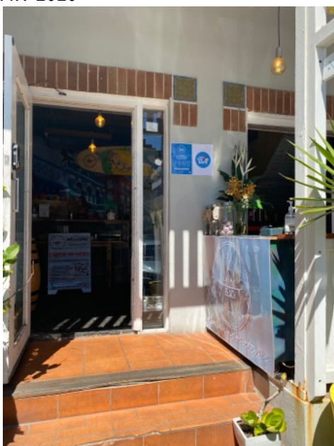
Figure 22.0, Shop opening to Victoria Parade, AW 2020
