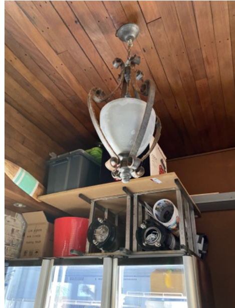
Figure 25.0, Timber lined ceiling, AW 2020
