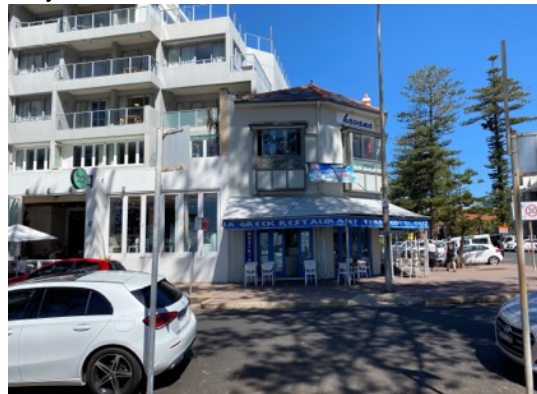
Figure 17.0, Corner Victoria Pde and South Steyne, AW 2020
