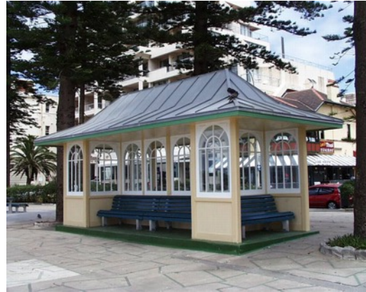
Figure 44.0, Public Shelter's (2) Federation. South Steyne. Environment NSW
