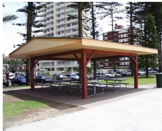
Figure 46.0, 1920s Shelter. Restored. Opposite Denison Street towards North Steyne, Environment NSW
