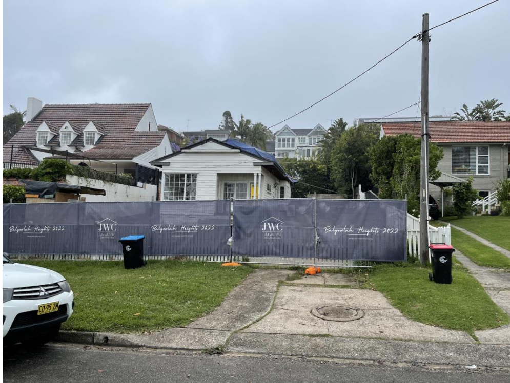
Fig 2: View of subject site and current access driveway, looking south-west from Beatty Street and towards the neighbouring dwelling to the south at No 9 Beatty Street
