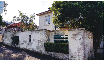
CONDITION OF FRONT FENCE
