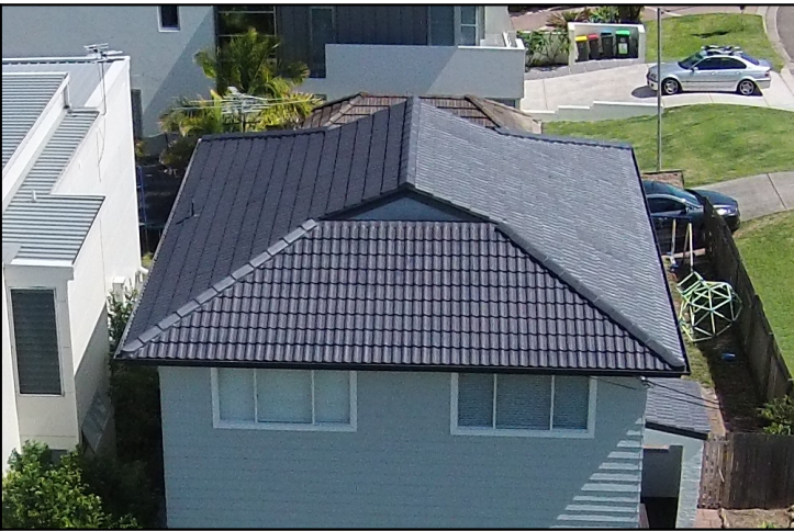
TILED ROOF & DUTCH GABLE TO MATCH EXISTING
