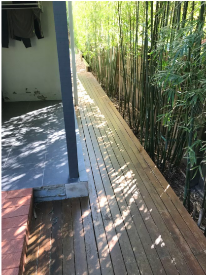
Fig.04 – Northern rear side access
