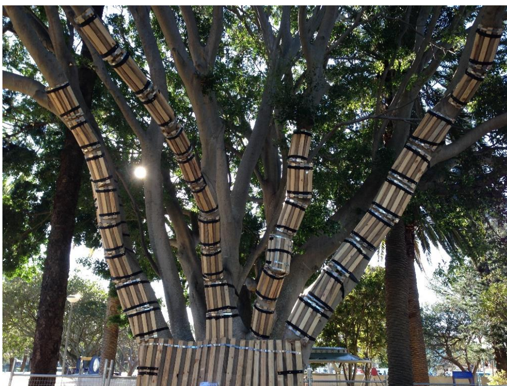
An Example of completed Stem Protection
