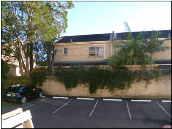
PHOTOGRAPH LOCATION 3 17-19 FORESTVILLE AVE
