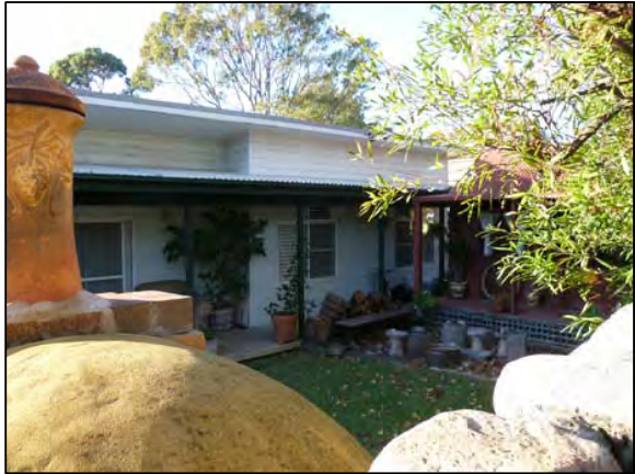
PHOTOGRAPH LOCATION 12 No.31 MELWOOD AVE
