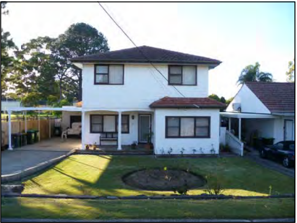
PHOTOGRAPH LOCATION 7 No.23 MELWOOD AVE
