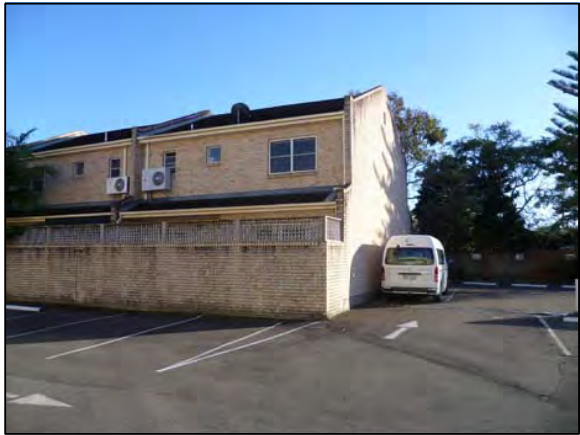
PHOTOGRAPH LOCATION 4 17-19 FORESTVILLE AVE
