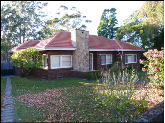
PHOTOGRAPH LOCATION 16 No.37 MELWOOD AVE
