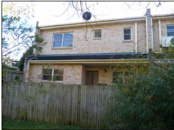
PHOTOGRAPH LOCATION 1 17-19 FORESTVILLE AVE
