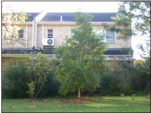
PHOTOGRAPH LOCATION 2 17-19 FORESTVILLE AVE
