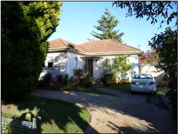
PHOTOGRAPH LOCATION 6 No.18 MELWOOD AVE
