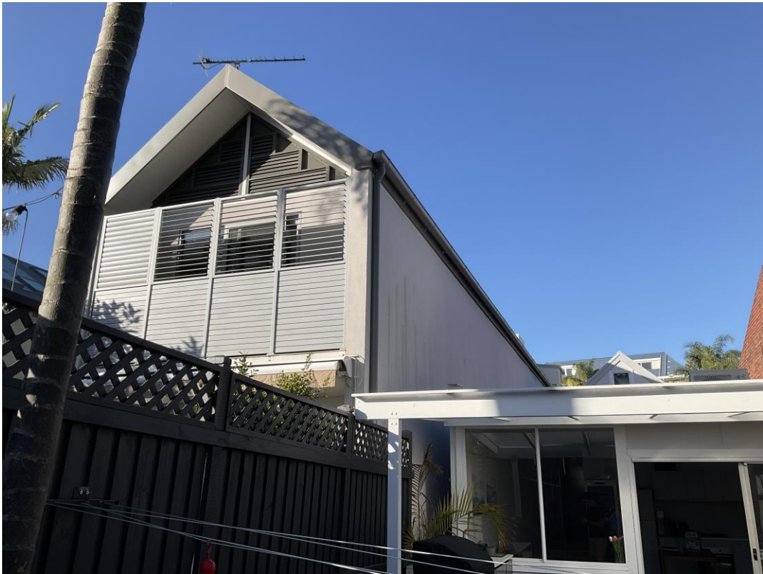
Figure 7. The neighbouring property to the north, looking northeast.
