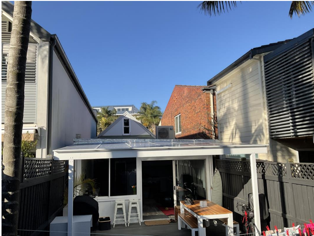
Figure 5. The rear of the dwelling, looking east towards Whistler Street.
