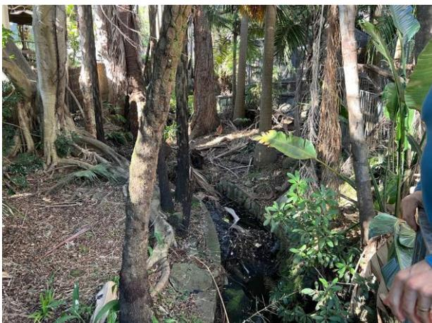
Plate 5. Existing drainage line with hard surface, concrete and rock lined in this upper section. Area covered by Waterway Impact Statement. This is marked as a first order creek on the NSW hydroline.
