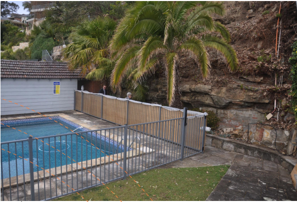
Existing Pool terrace and fencing
