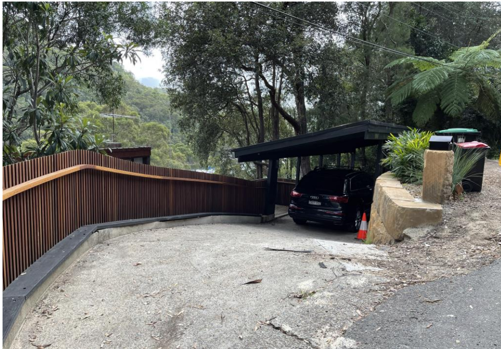
Figure 4: The existing driveway and carport, looking north from McCarrs Creek Road.
