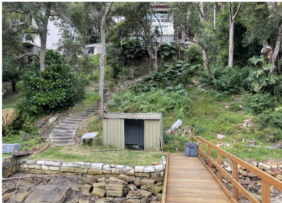
Figure 5: The seawall, jetty, disused neighbouring inclinator and rear of the site, looking east.
