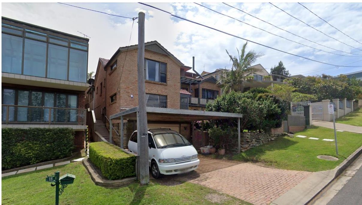
Figure 3: Subject site as viewed from Taylor Street (Google Maps 2023)
