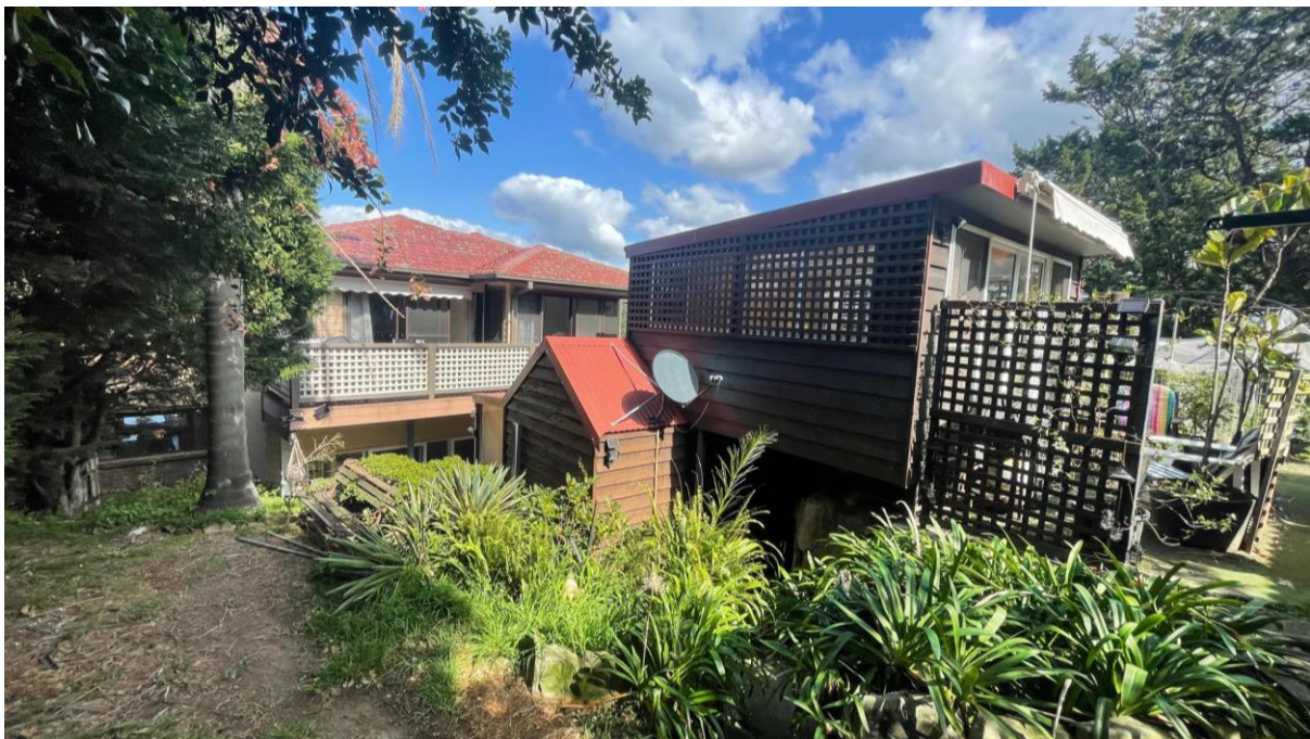
Figure 5: Two-storey building in the rear yard (Corona Projects 2023)
