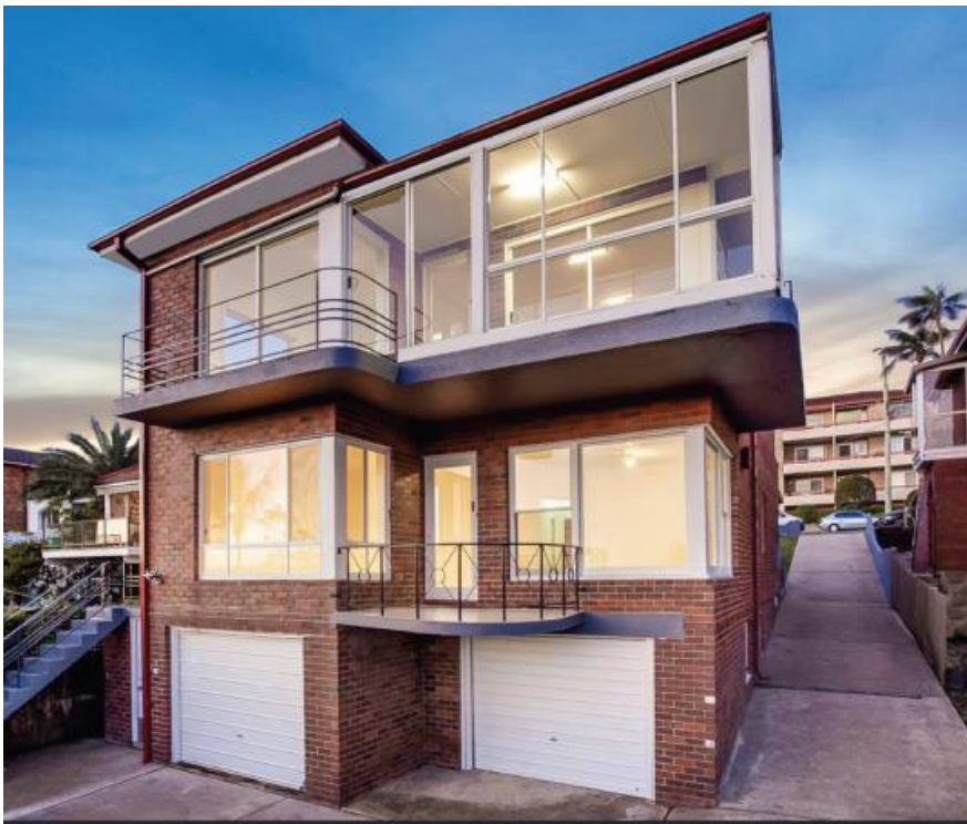
Figure 4 - the existing 3 storey character to the rear at 124 Queenscliff Road as viewed from the south-east
