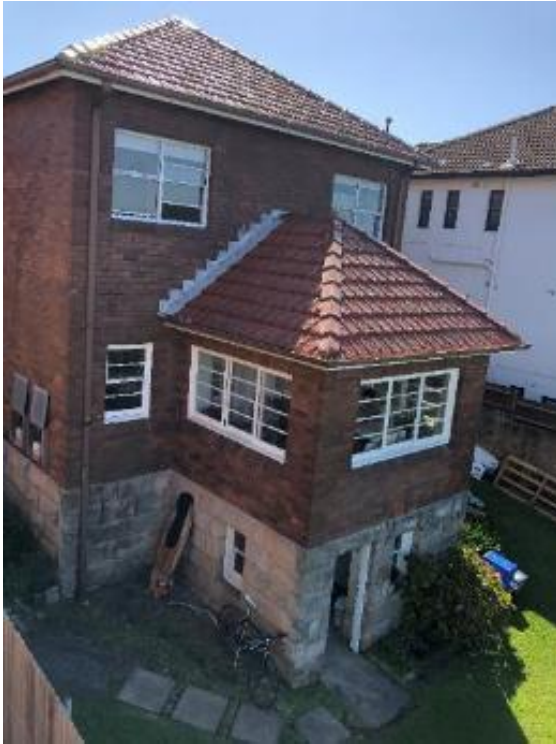
Figure 3 – the existing 3 storey character to the rear of 122 Queenscliff Road
