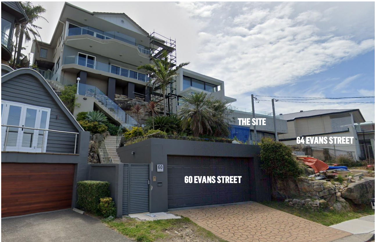
View 5 – View north-east towards the site from Evans St. with No. 60 in the foreground.
