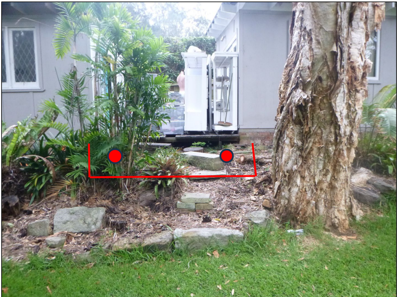
Photo C: Area where test digging is required to determine pier footing locations.
