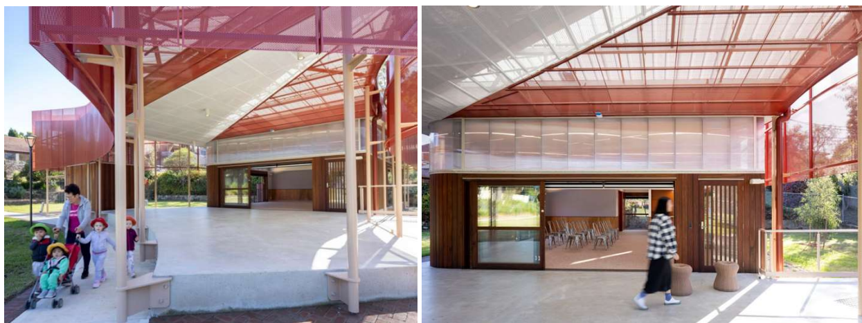
Photo 7.1 Hurlstone Park Community Centre (Sam Crawford Architects) located in Hurlstone Memorial Reserve Park Source: https://www.architectureanddesign.com.au/projects/cultural-entertainment-sports/hurlstone-park-community-centre-sca
