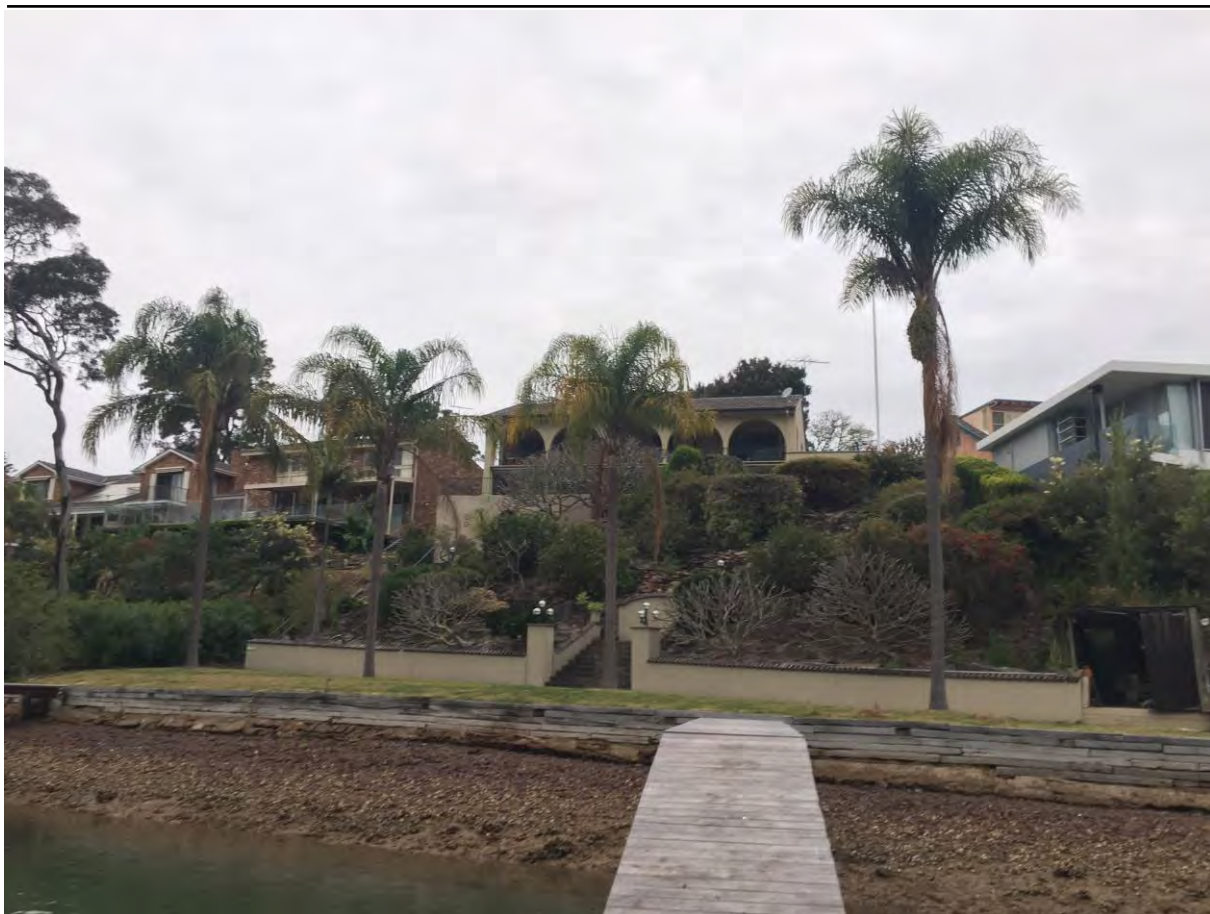
Figure 6 Sea Wall at foreshore of 3 Panima Place, (retaining wall to rear of grassed area). captured 30 September 2015
