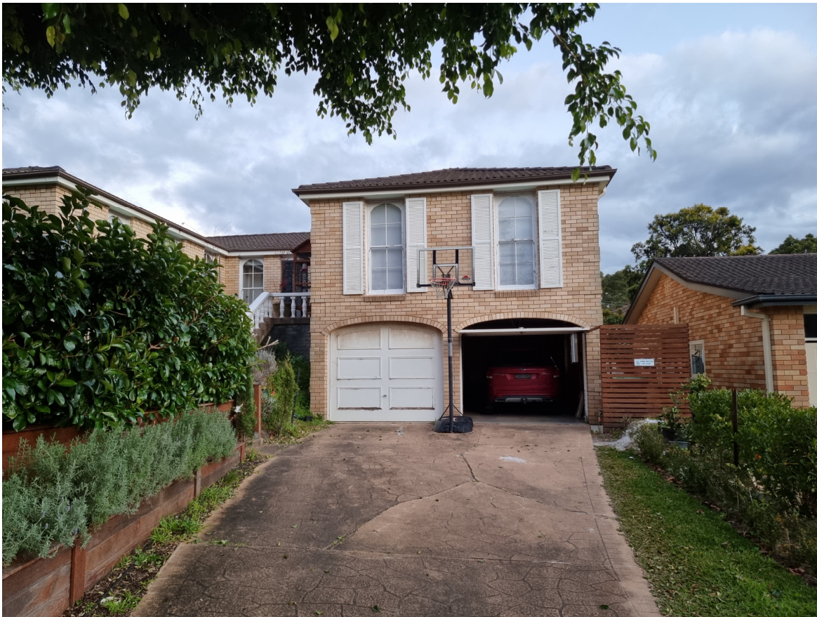
View of the existing garage
