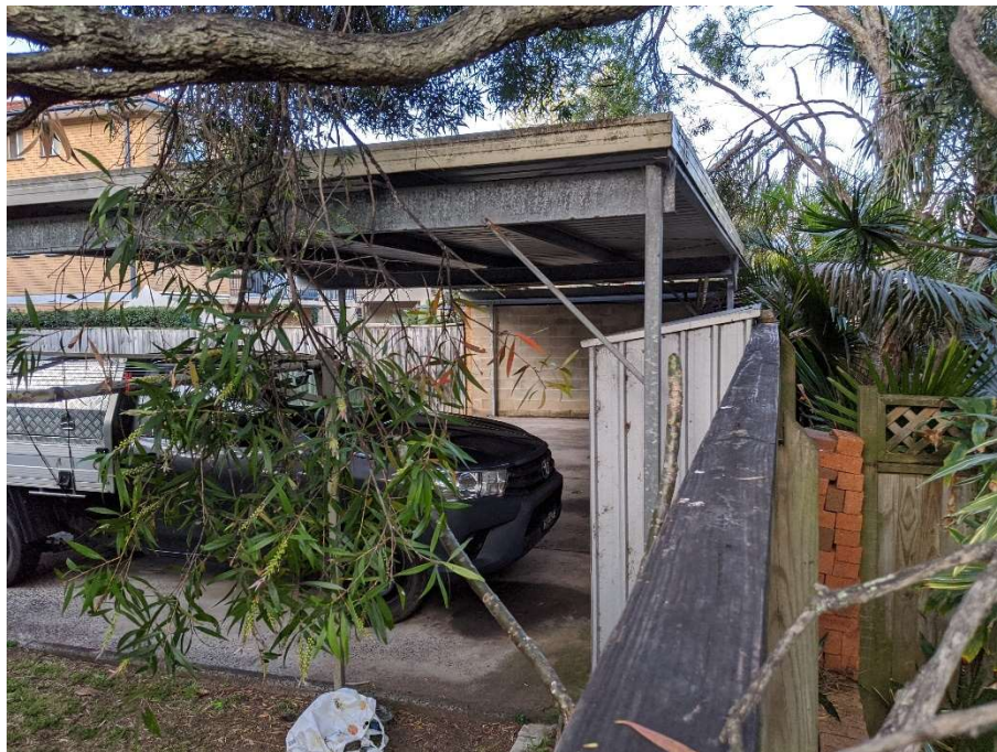
Figure 11: Carports to rear of site
