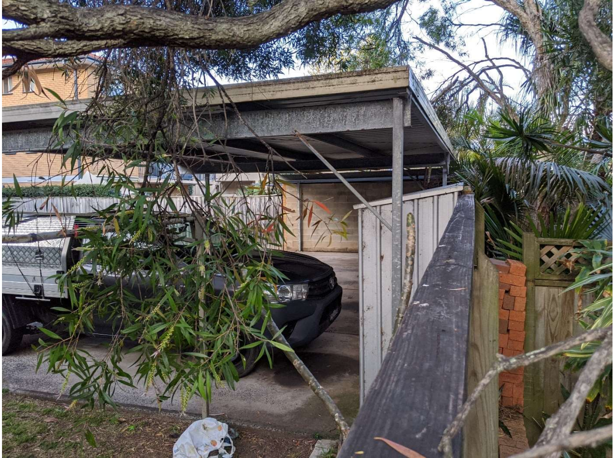
Figure 7: Boundary fence interface at northern boundary showing carports immediately to north of subject rear open space area.
