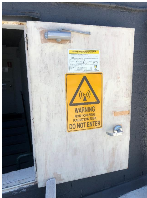
Figure 7 – Access restriction and EME Warning Sign
