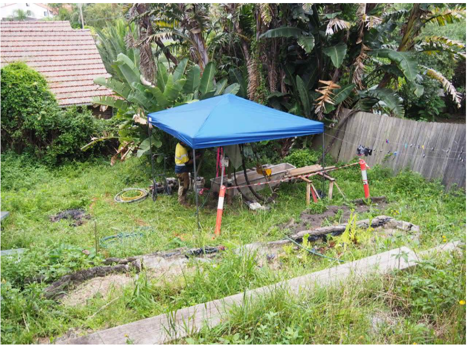
Photo 3 - Drilling Bore 3 on 31 Reddall Street
