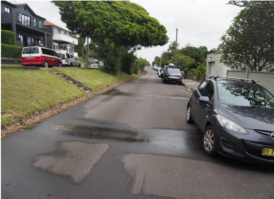
Photo 6: Seepage across Reddall Street following extended rainfall
