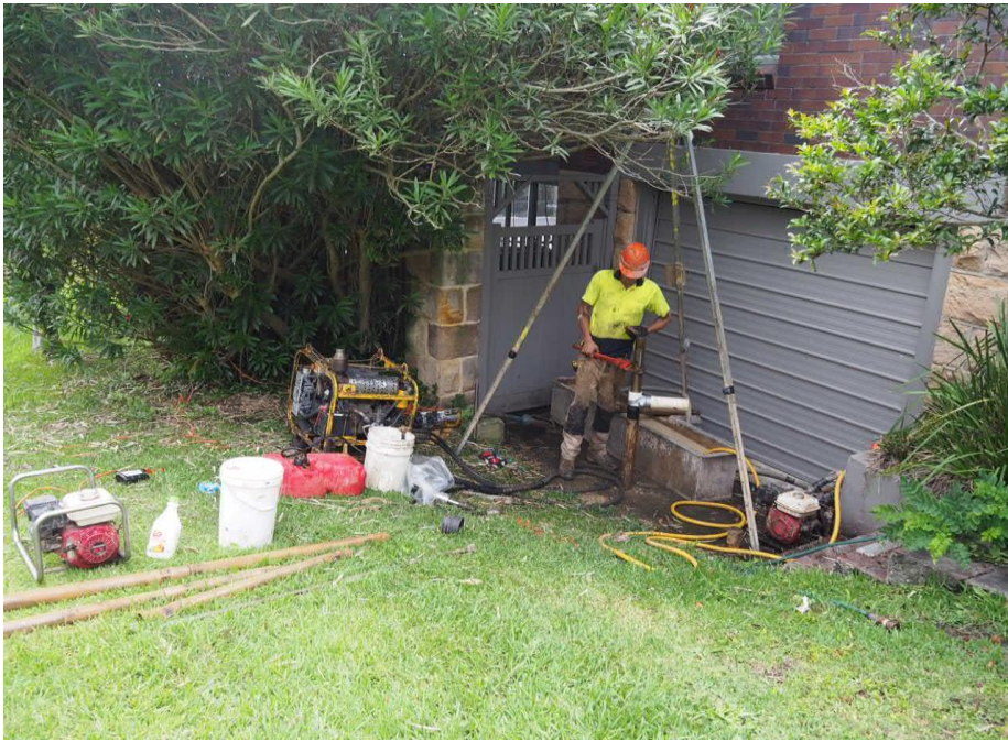
Photo 1: Drilling Bore 1 on 29 Reddall Street
