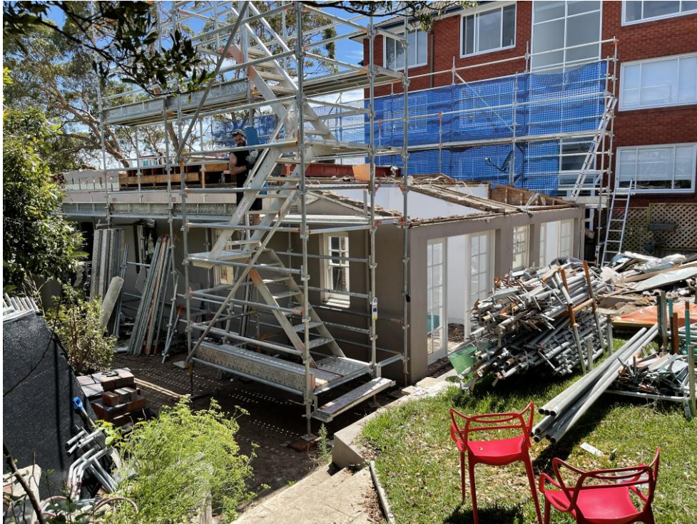
Fig 4: View of the existing dwelling undergoing additions alterations in accordance with the recent development consent and location of the proposed swimming pool in the LHS foreground
