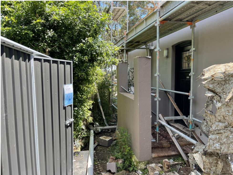
Fig 5: View looking north along the western boundary and the location of the proposed swimming pool adjacent to the western boundary adjoining public walkway
