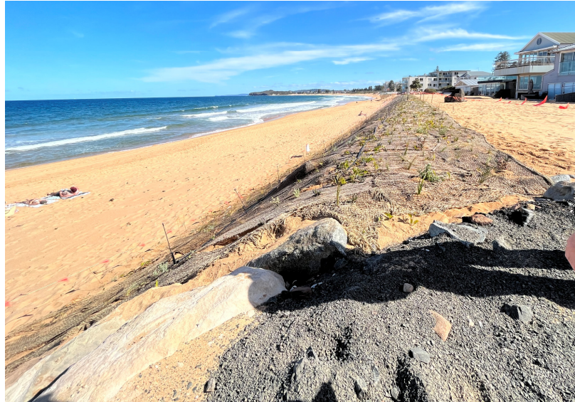
Figures 9 and 10 – Completed revetment wall (Jan 2023)
