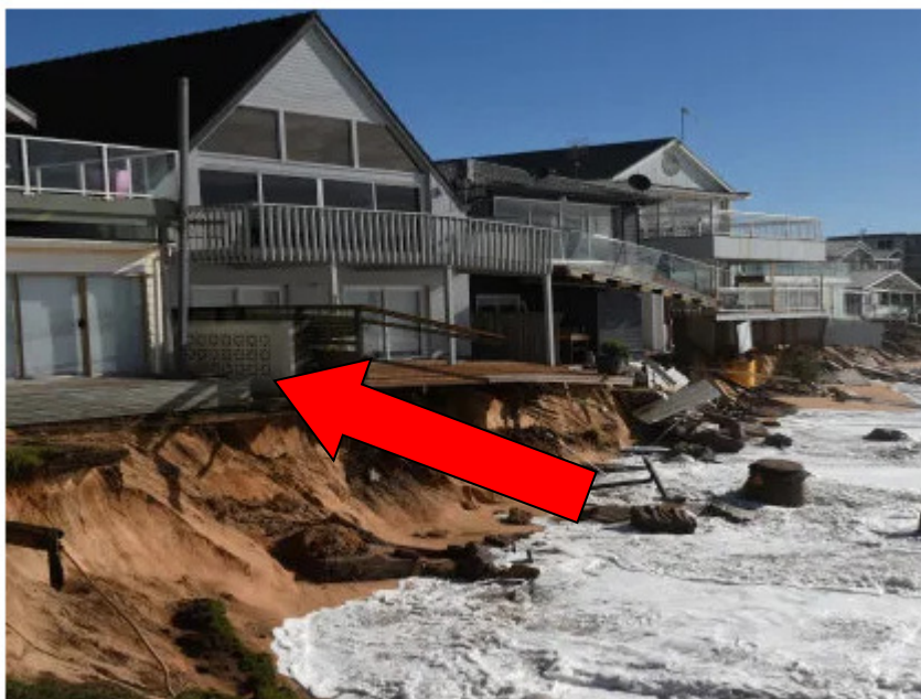
Figure 8 Photo of eroded east side of subject site taken in 2016.
