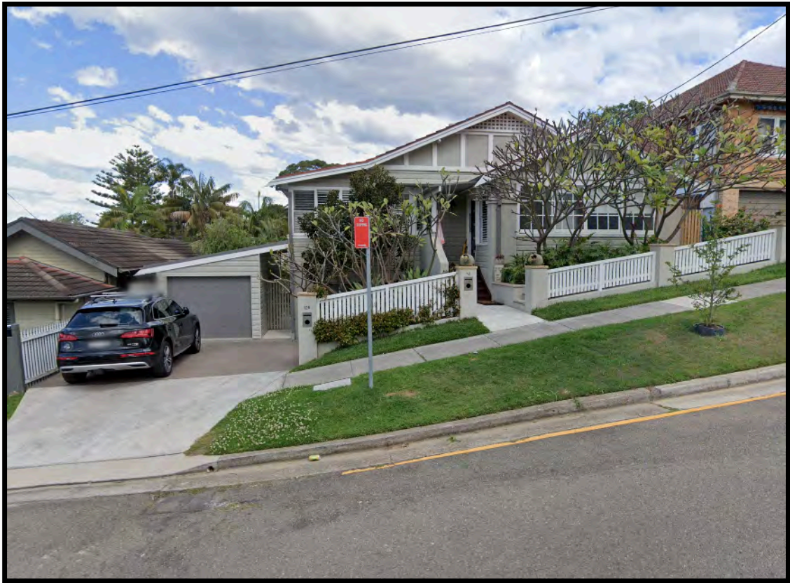
Image 2 – Streetscape and 12 Collaroy Street
