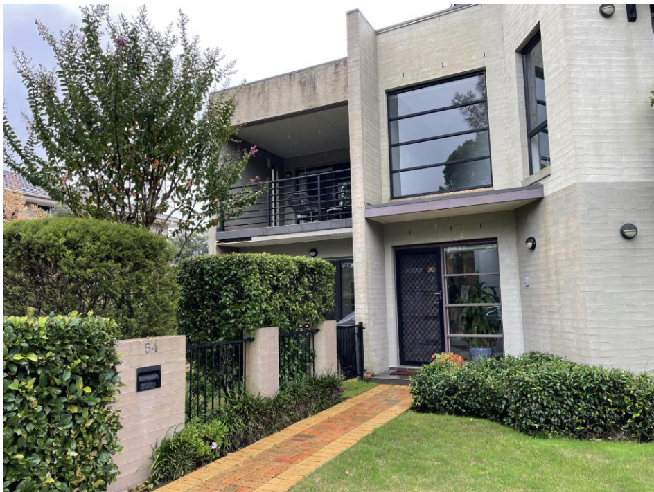
Figure 7: The existing front of the dwelling and location of the balcony.
