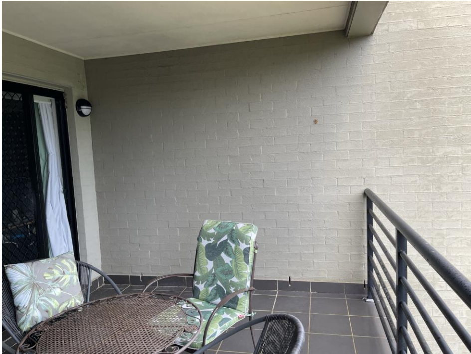
Figure 8: The existing balcony.
