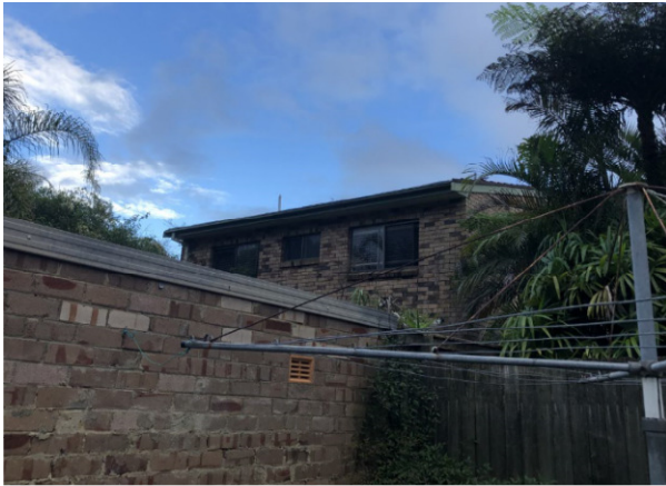
Photo 3- View of 3/2 Bolingbroke Parade
