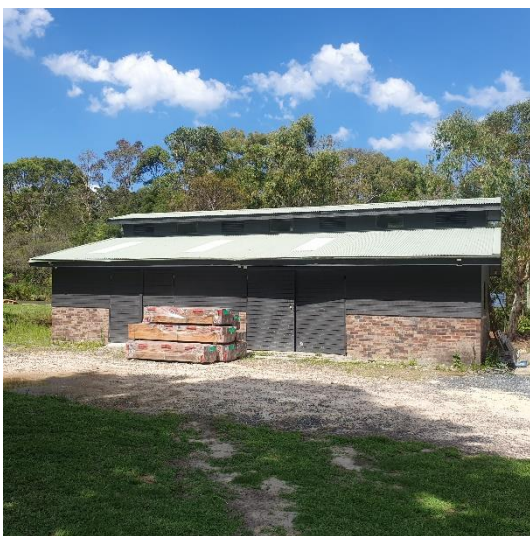
Photograph-1: The barn. View looking east.
