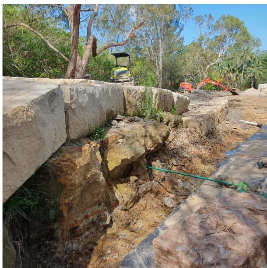
Photograph-4: Residual material/EW bedrock. View looking east.
