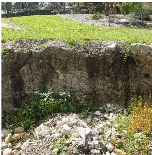
Photograph-2: Excavated bedrock. View looking north.
