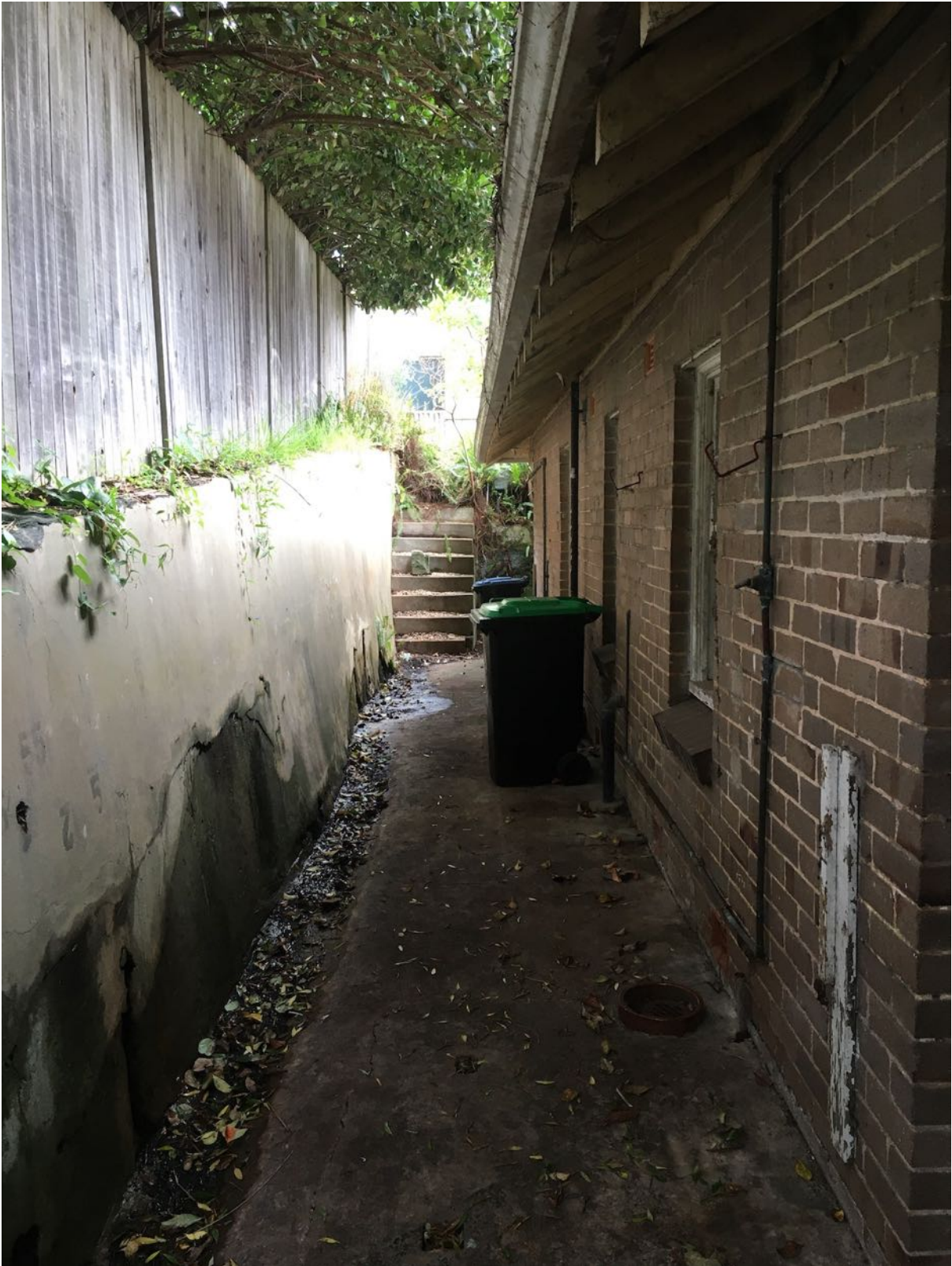
Figure 1. Back of the house looking to western boundary, showing the retaining wall and stairs to be removed at far end
