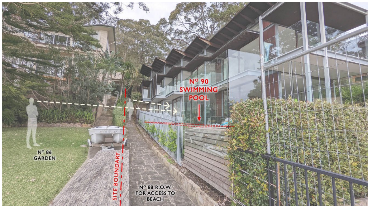
FIG. 10 – EXISTING NORTHERN BOUNDARY & POOL PRIVACY ISSUES
