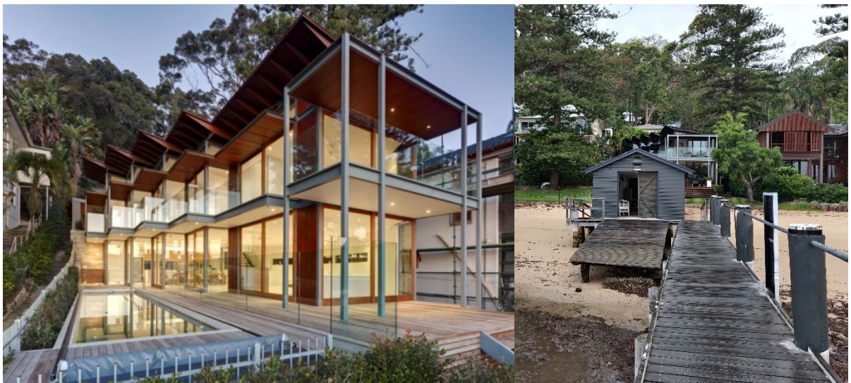
FIG. 2 VIEW OF EXISTING HOUSE & BOATHOUSE FROM PITTWATER
