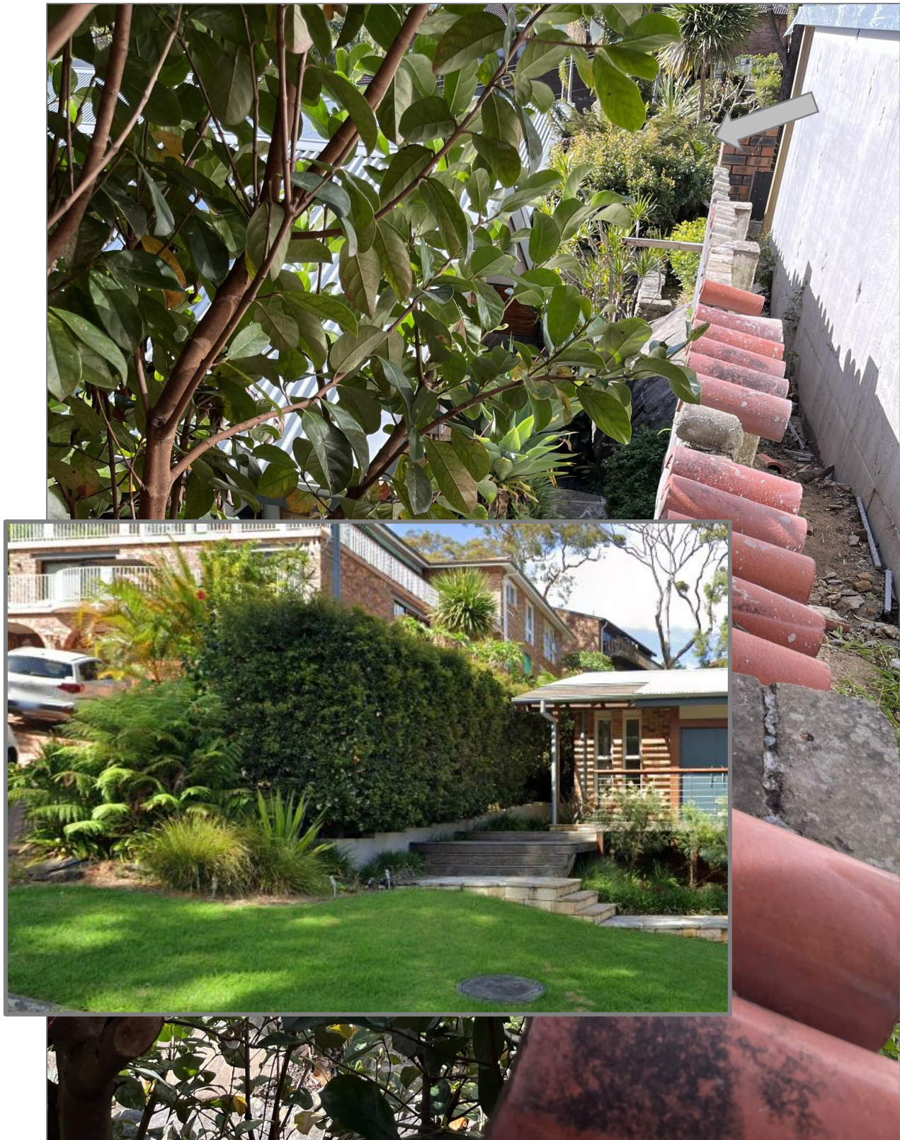
Plate 5 – Group 3 – Arrow notes hedge, not assessed at time of inspection as was not in scope at that time. INSET – street view of hedge taken from Google Maps.
