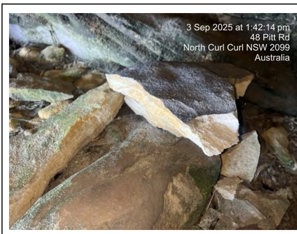
Photo 5: Evidence of recent localised failure.
