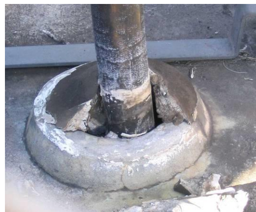
Figure 19 – Asbestos cable tape in substation and broken NC compound
