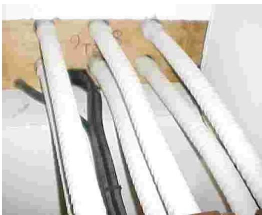
Figure 19 – Asbestos cable tape in substation and broken NC compound
