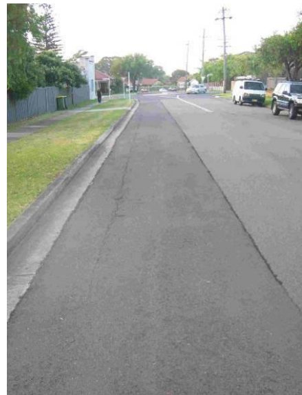
Figure 12 – Permanent reinstatement
