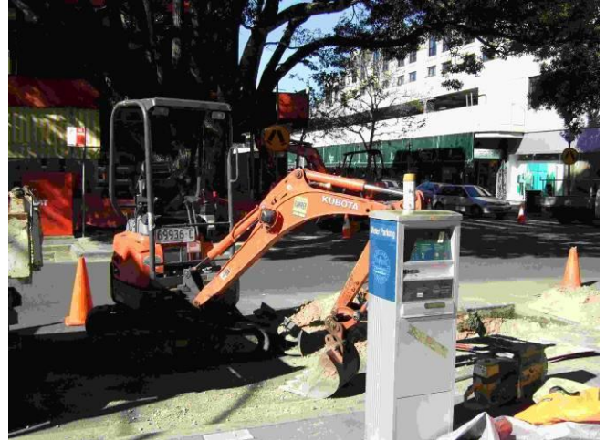
Figure 9 – Excavation and removal of sub-surface material
