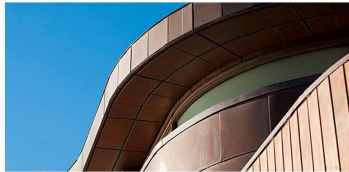
G - COPPER STYLE ROOFING
