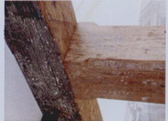
EXPOSED TIMBER INTERNALLY AND EXTERNALLY
