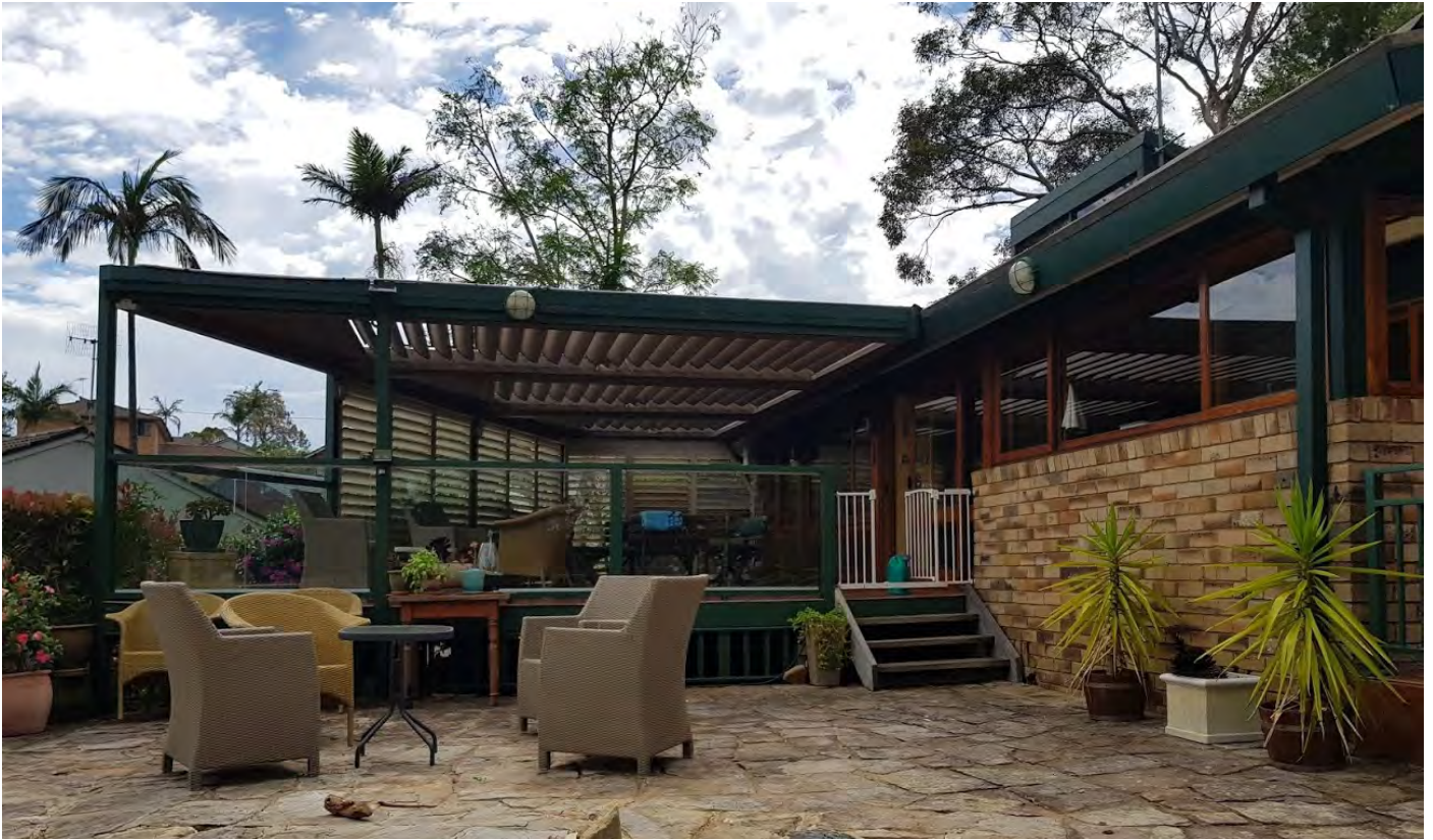
5. Photo of the existing.
