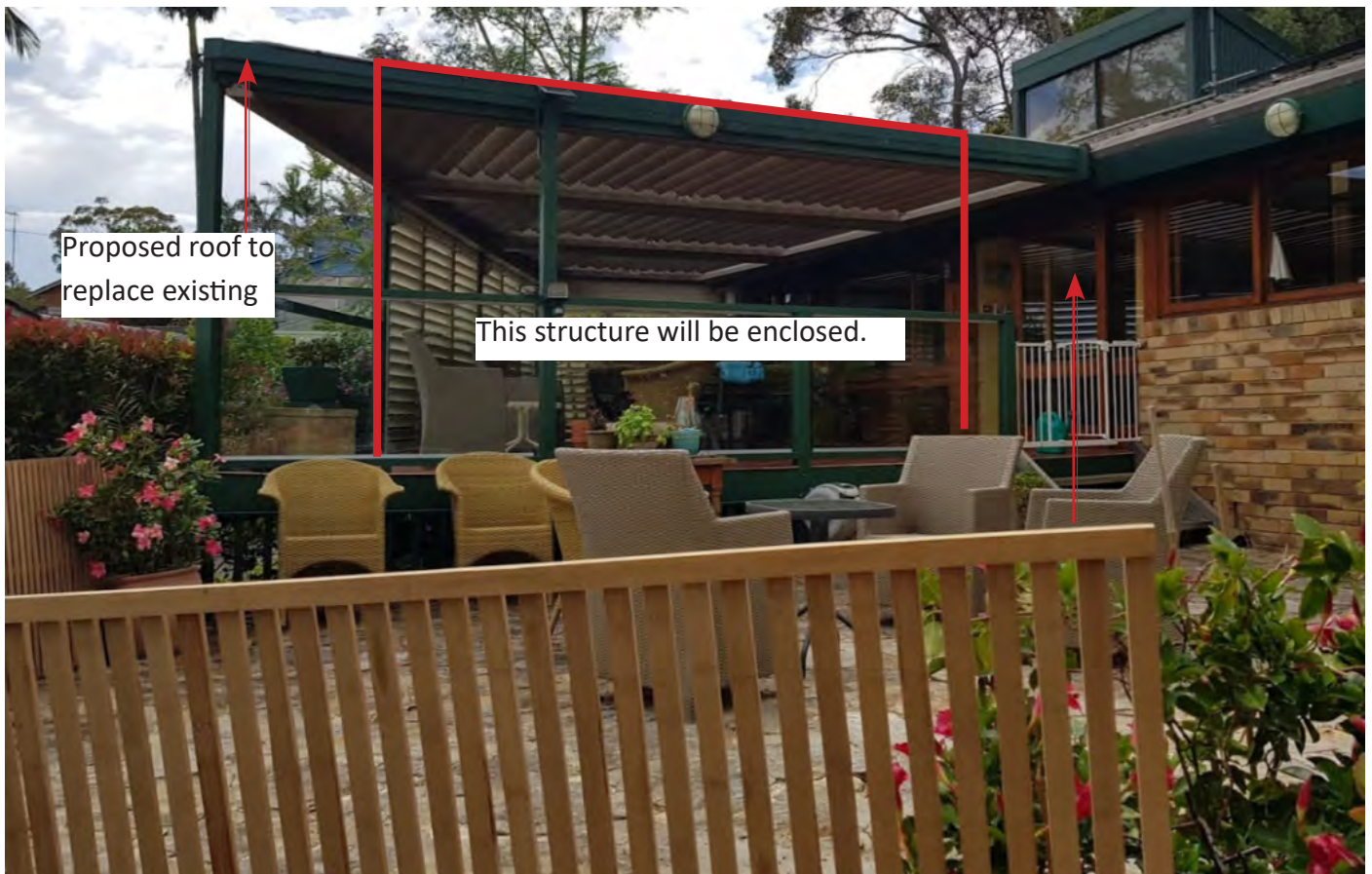
Photo 1 - View looking east towards the structure to be replaced.
