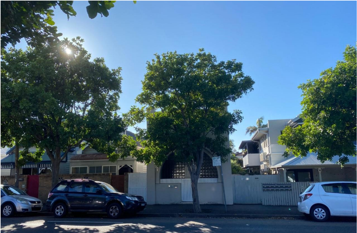
Photograph of the subject site – 122 Pittwater Road, Manly – the front façade is unique and different to other dwellings along the street.
