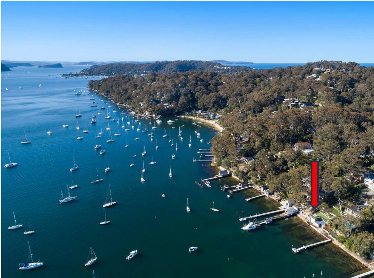
27 Riverview Road boatshed rooftop terrace overhead view
