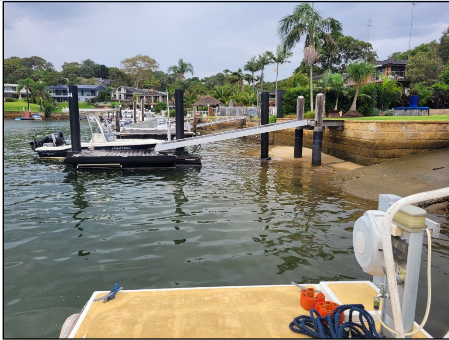
Figure 5 – southern neighbours' facility
