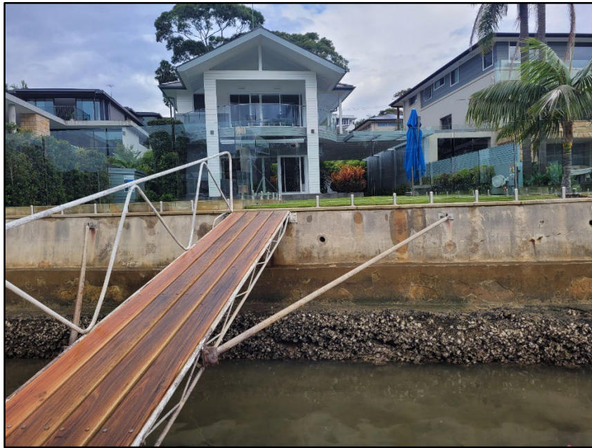
Figure 3 – attachment of timber ramp to seawall
