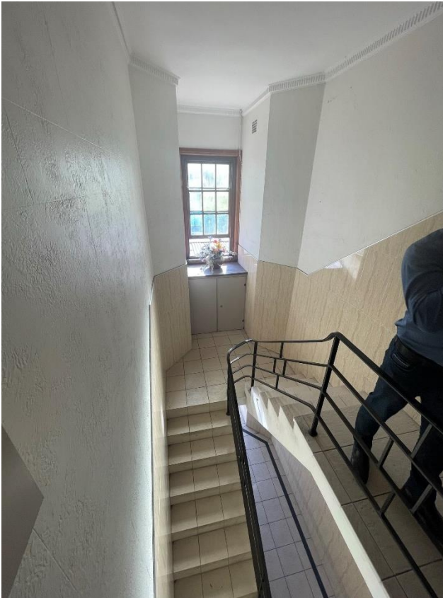
Figure 38 – Upper landing of central stair Source: Urbis, March 2023
