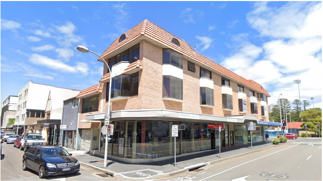
Figure 48 – 42-43 Belgrave Street, east façade as viewed from intersection of Raglan & Whistler Streets Source: Google Maps, 2020
