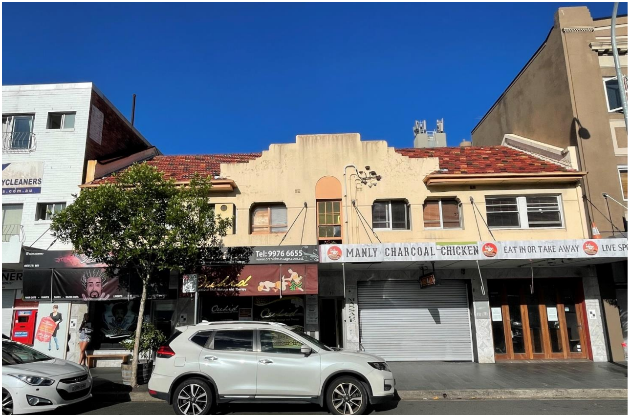
Figure 32 – 35-39 Belgrave Street, principal elevation at Belgrave Street Source: Urbis, March 2023
