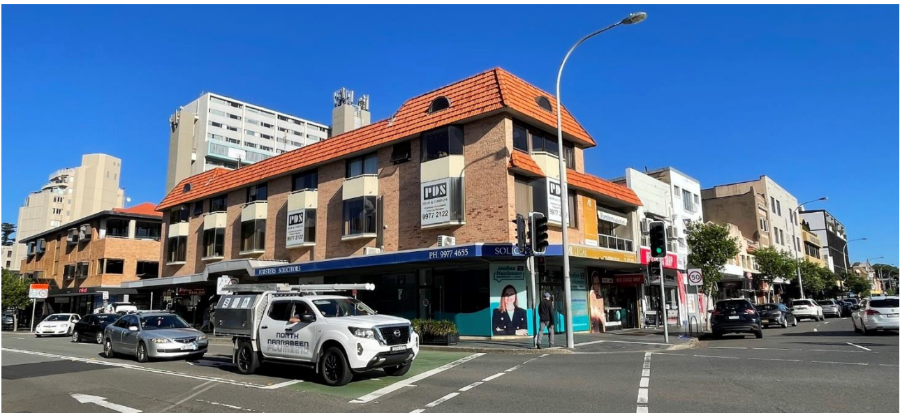
Figure 47 – 42-43 Belgrave Street, north façade as viewed from intersection of Belgrave & Raglan Streets Source: Urbis, March 2023
