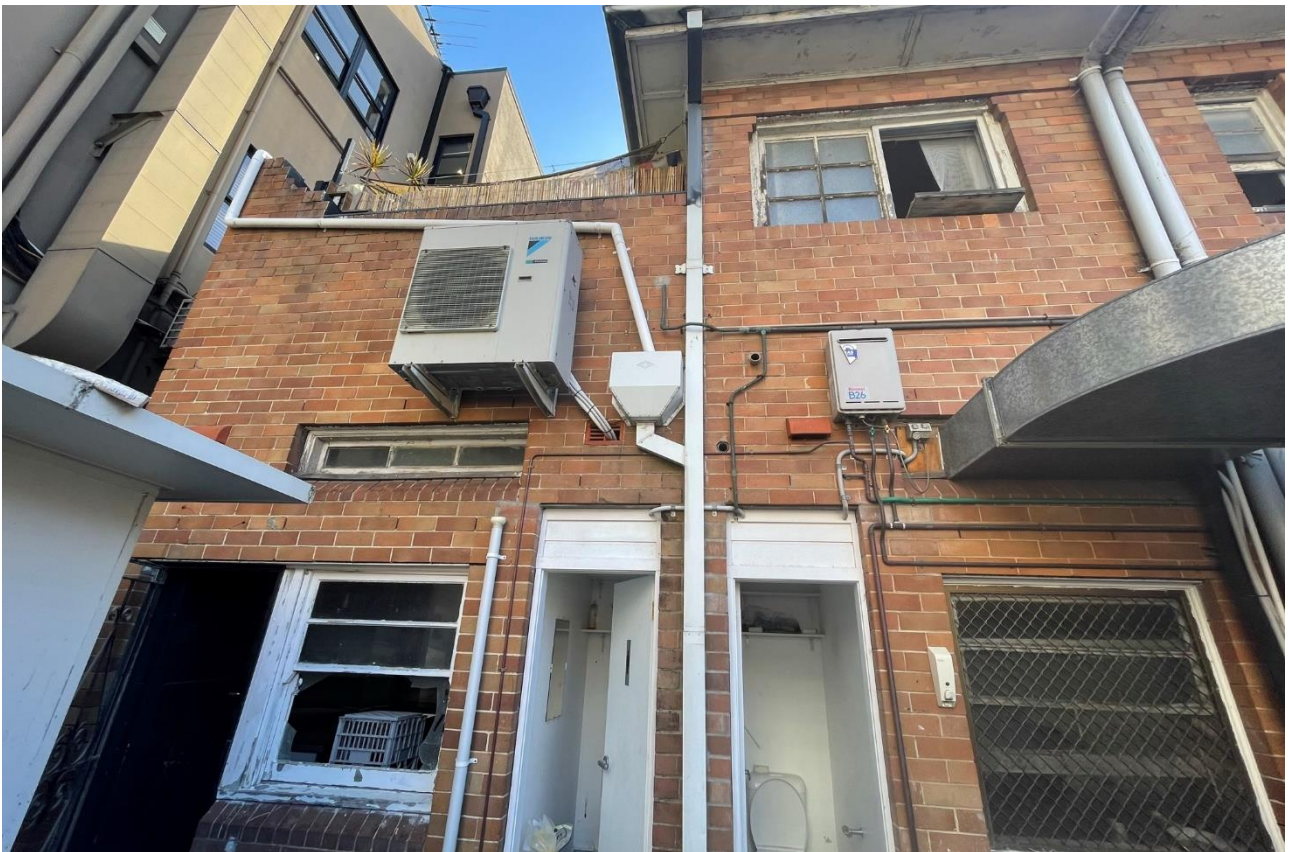
Figure 34 – Detail of rear elevation of 35-39 Belgrave Street Source: Urbis, March 2023
