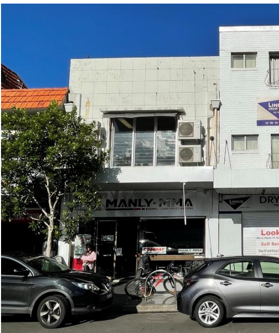
Figure 44 – 41 Belgrave Street, west elevation at Belgrave Street
