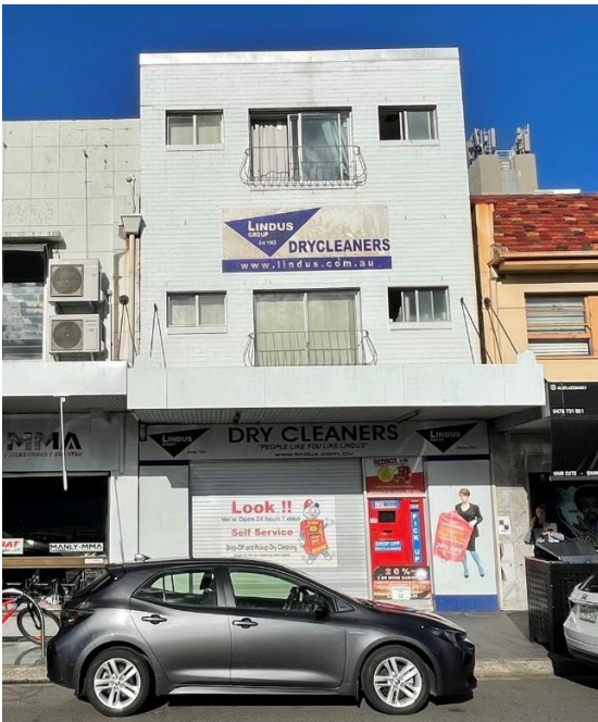
Figure 42 – 40 Belgrave Street, west elevation at Belgrave Street
