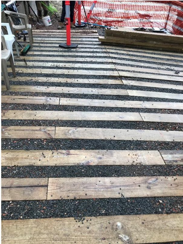
Figure 9 Sleepers with gravel between protecting ground from compaction
