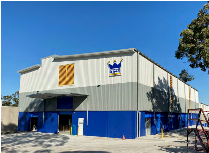
VIEW OF BUILDING 2
