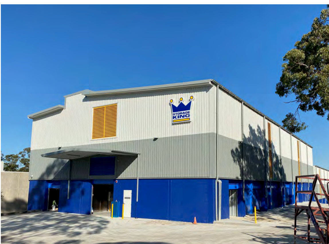
VIEW OF BUILDING 2 SHOWING EXISTING SIGNAGE
