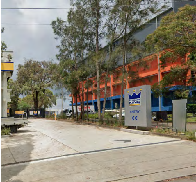
VIEW OF EXISTING PYLON SIGN
