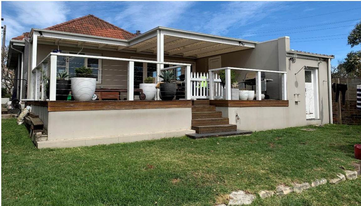
Photograph 2. View of the rear of the main structure, facing south
