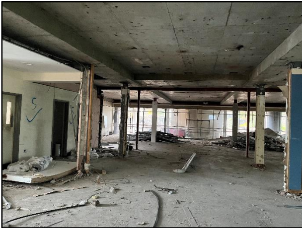
Figure 22. Internal view of the lower ground floor of Building 6, facing south showing the base build works in progress. Note the later-addition office fit-out has been removed.
