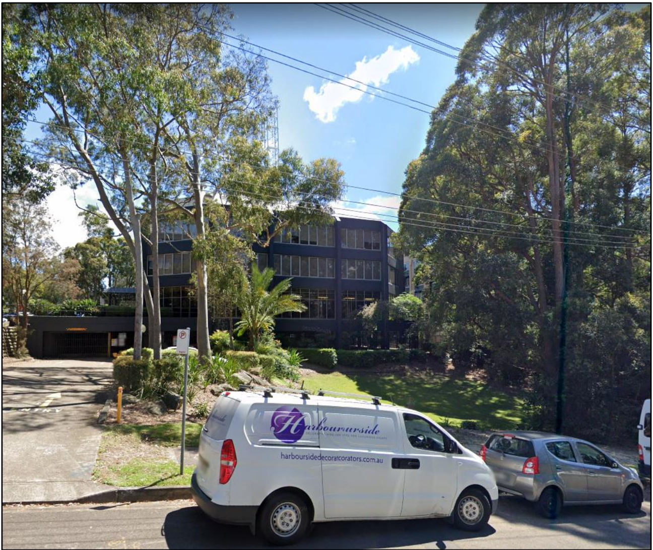
Figure 3. View north from Rodborough Road, towards the existing building at the Site (Google Street View, 2021)
